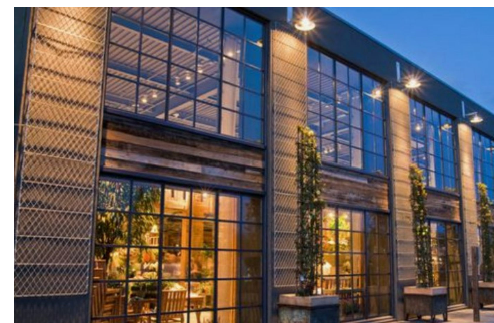
STEEL SCREEN OVER EXTERIOR PAINTED CMU OPTIONS
